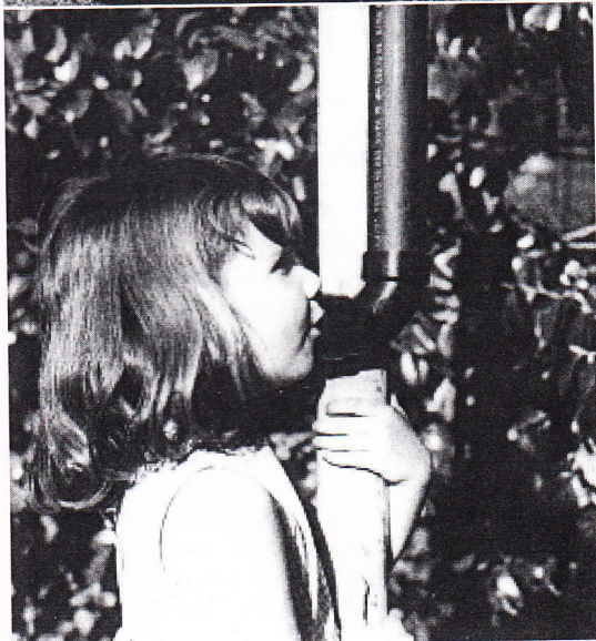
Voice tube made from PVC tube and brass snap-strainer connects three levels of the Hide Away, Human Resources Centre, Pontiac, Michigan. Voice tube adds a variable to any structure, allows experiments in communication, increases perception of space and volume.
